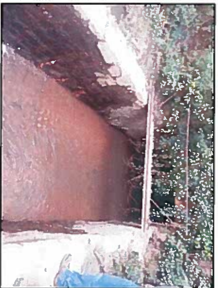
South Culvert: 10'x7' RCB with weir control structure at inlet
