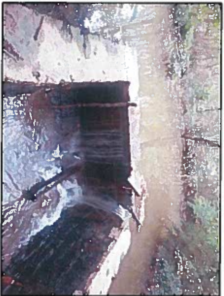
South Culvert: 10'x7' RCB with weir control structure at inlet
