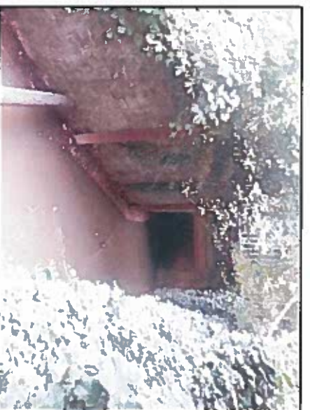
South Culvert: 10'x7' RCB with weir control structure at inlet
