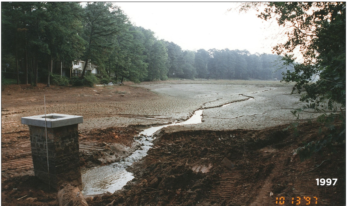
View from the new dam with the lake drained in 1997. The entire area shown in this picture has never been dredged. Sediment has increased over two feet since this picture was taken.
